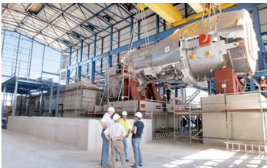
Weighing in at 444 tons, the world's largest turbine is carefully positioned.
